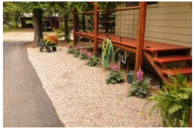
Upper Level Driveway & Deck
