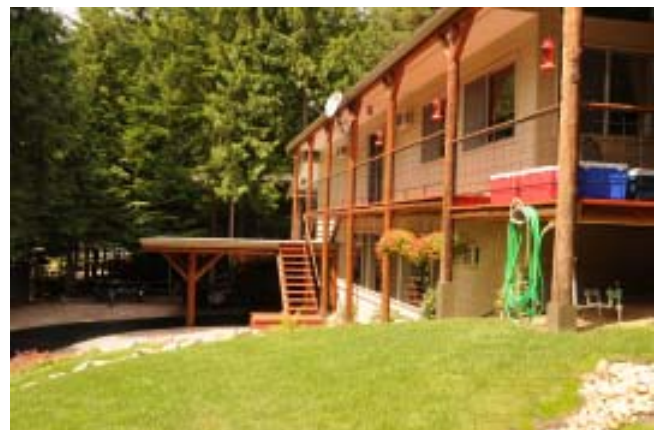
Street View of Lower Level
