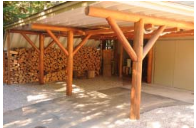
Lower Carports & Wood Storage
