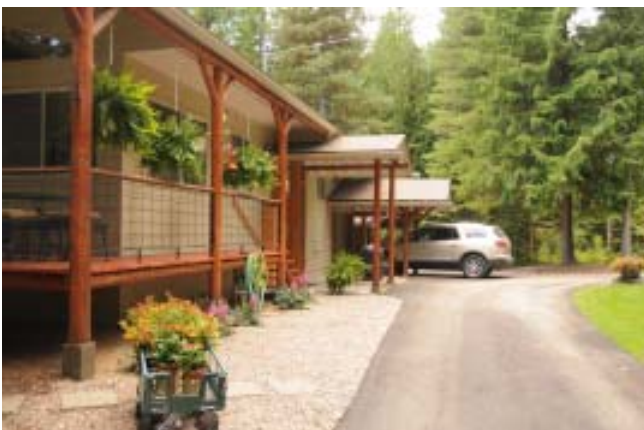
Upper Level Driveway
