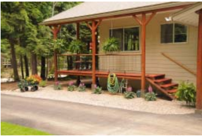
Upper Level Driveway & Deck
