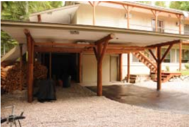
Lower Level Carports & Garage
