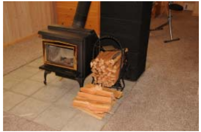
Lower Level Wood Stove
